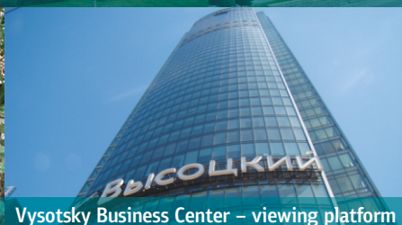
Vysotsky Business Center – viewing platform
